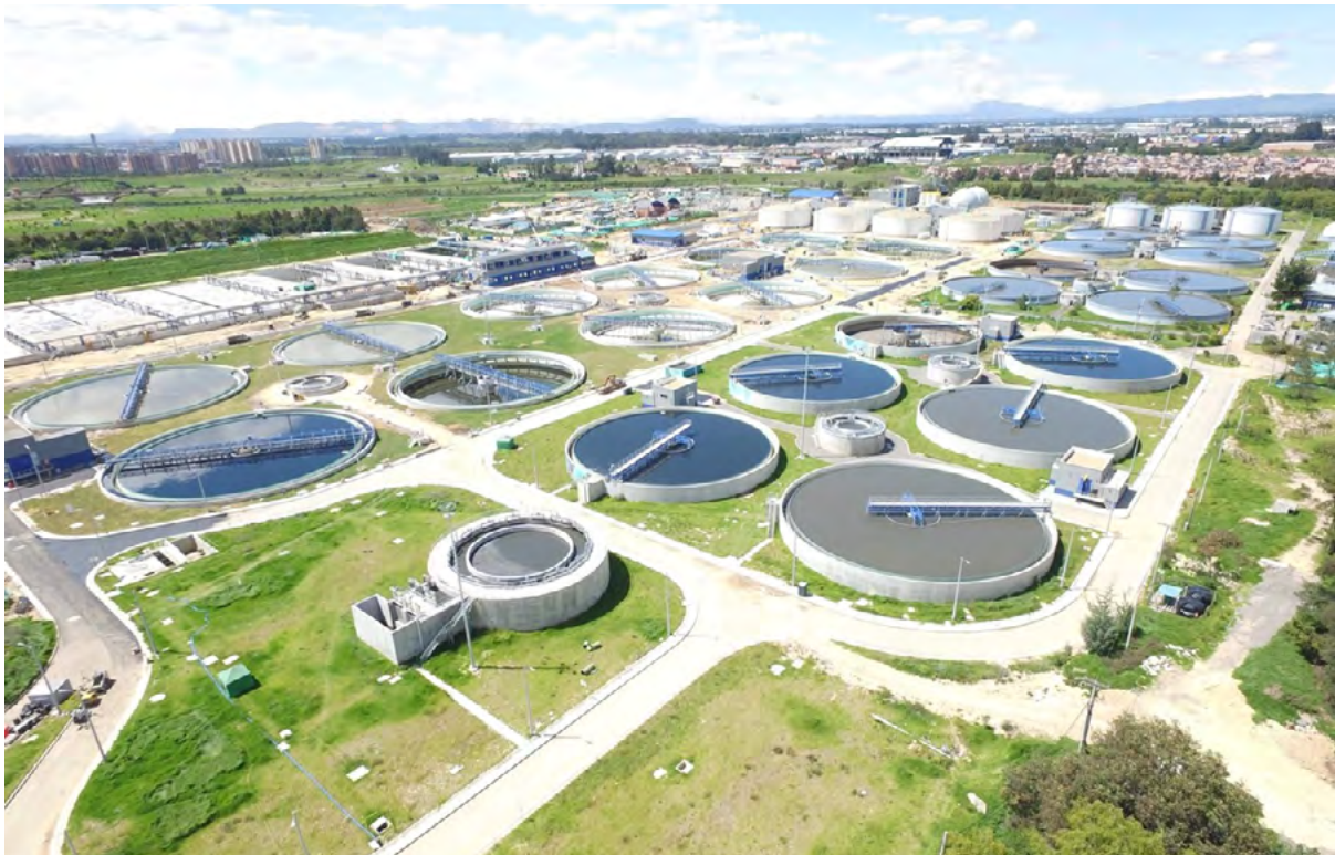
Figure 4. Progress at the Salitre WWTP in 2021
